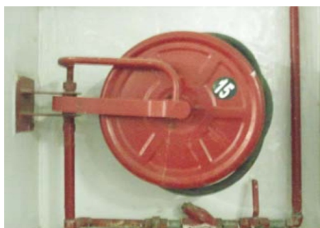
Fig. 7.6.2.1: Kaizen Before – Used for single department – Front of the wall
